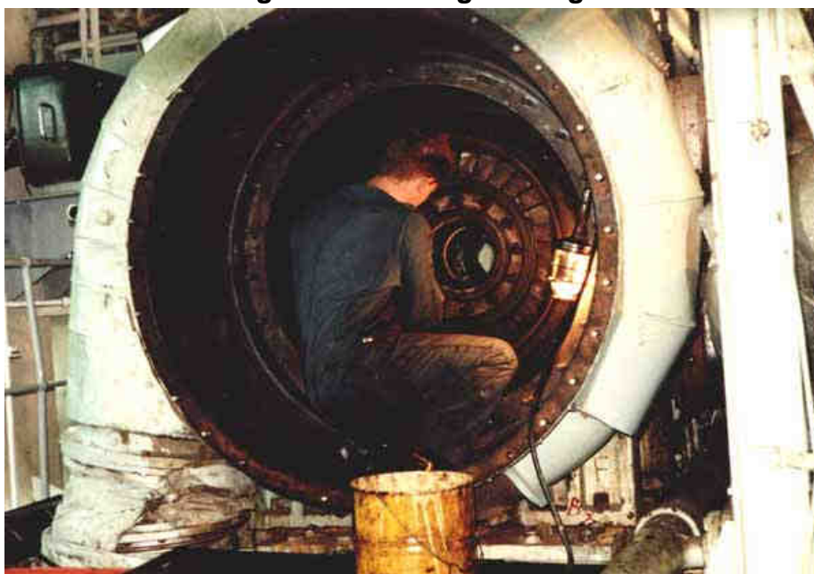
A main engine turbocharger being serviced
