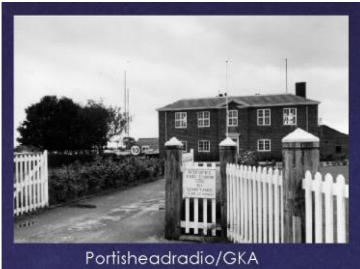
British Post Office station Portishead Radio
